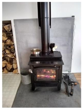
I cleaned the woodstove with a wire brush and repainted it with high temperature enamel. We will likely paint the heat shields in the spring when we can take them outside to spray. At that time, I will also move the floor panel and insulation panel below it over about 3 inches to align with the one on the wall.
