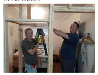
After a day of adding a number of new outlets and running a few more lines to the electrical panel, we insulated the place with R14 Roxul and added vapour barrier to the outside walls.
