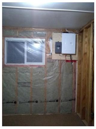
The fuse panel located in the second bedroom was removed and a new 100 amp breaker panel went in its place. The new wires we added now had separate breakers for each room.
