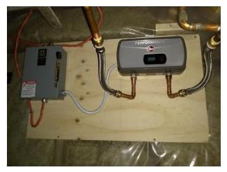
While we were there, the old water heater gave out, so I picked up a point-of-use electric water heater and installed it near the bathroom, ensuring warm showers and handwashing.
