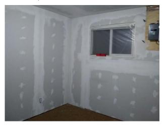
Dry-walling continued in the other rooms as I taped, filled and sanded all of the joints in preparation of painting the walls and ceilings throughout the cottage.
