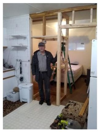
With Lee there we were able to get a photo or two of Rob and I working too. The framing was to inset the refrigerator into the wall to make more room in the main living area and open it up a bit. We took about 2.5 square feet from the closet and 5 from an unusable corner of the main bedroom.
