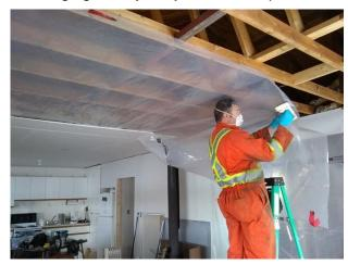
As with the exterior walls, we installed 6-mil vapour barrier over the joists before dry-walling the ceiling. The attic guy (Rob) then went up and installed the insulation between the joists and a second layer over it for good measure.
