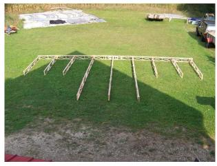
When Mike tested the flex in the main truss by hanging his body (approx. 170 lb.) from centre point while it was on saw horses, it only dipped about one inch. Not too bad for a 32 ft. span.
